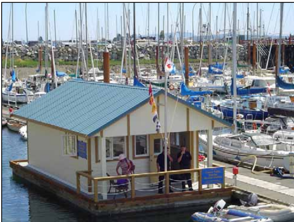
On January 13, 2007, Unit 60 Comox officially opened their new marine rescue station. The station provides a crew training/office area, maintenance, storage, and equipment drying area that is in close proximity to the unit's fast response rescue vessel Bruce Brown II. Photo Courtesy Brian Cameron
